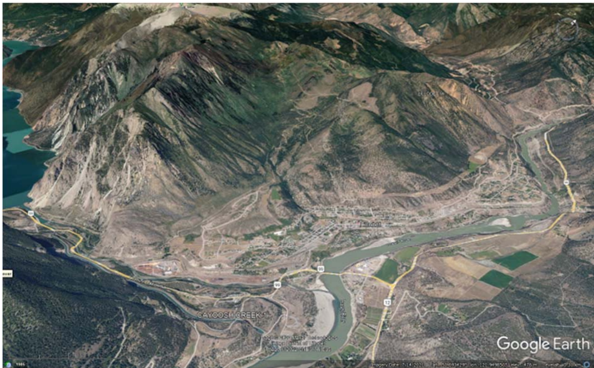
Figure 3.1 District of Lillooet – Aerial View from SE
