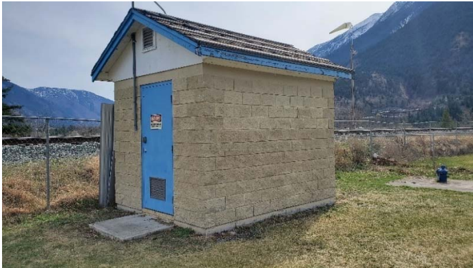
Conway Park Well No. 1 - South of controls building
