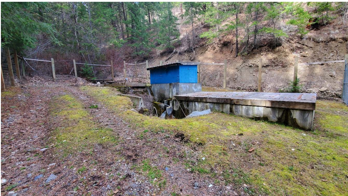
Photo – Town Creek Intake structure
