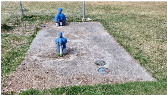
Conway Park Well 1 (150mm casing foreground) Conway Park Well 2 (250mm casing) further to west
