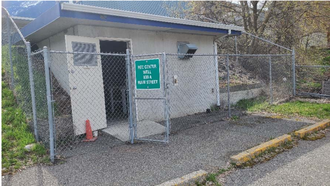
Recreation Centre Well Building Exterior
